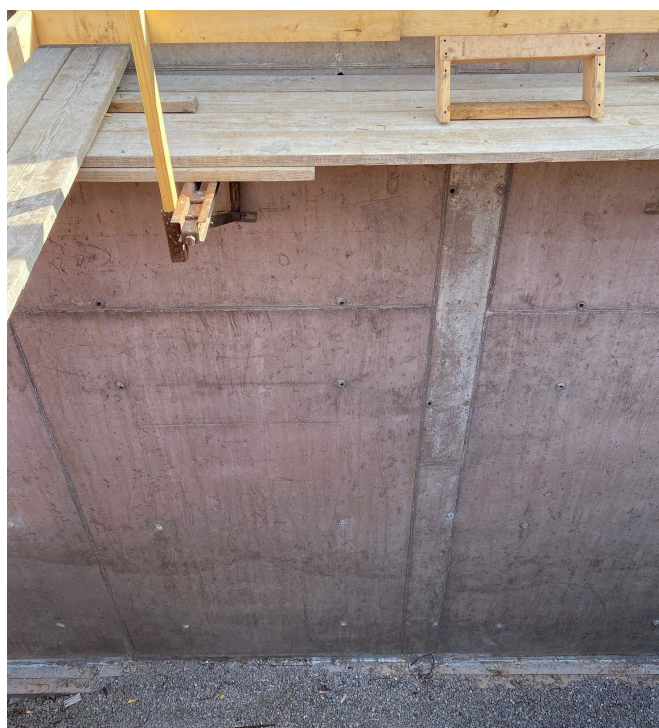
Xypex Bio-San was directly added to the concrete eliminating the need for a liner.
